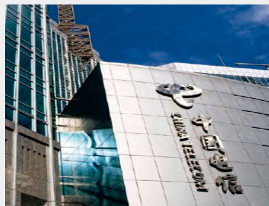
■ China Telecom Lingang Intelligent Computing Valley
