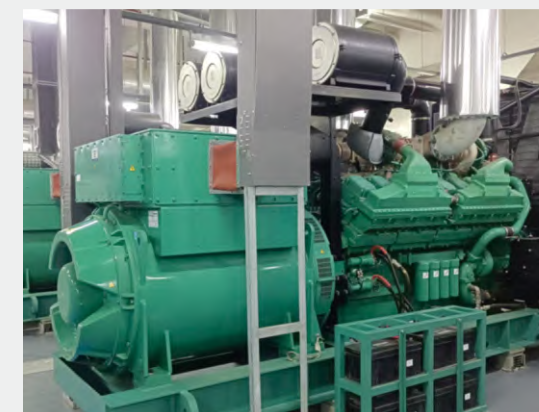
■ China Telecom Inner Mongolia Information Park
